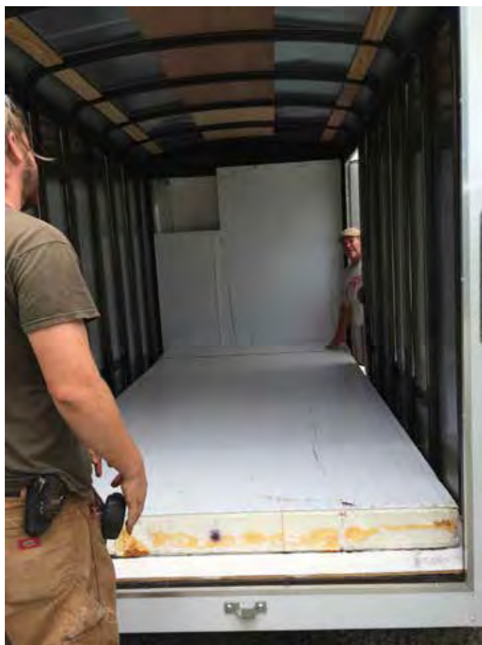
Figure 4. Set the front wall and floor first. The opening at the front should be wide enough to fit the air conditioner unit, 6 inches of insulation, and any airspace outside the insulation.
