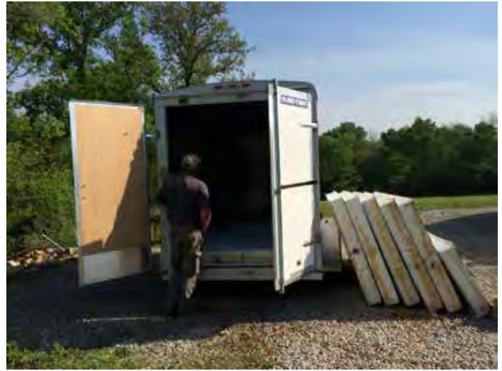
Figure 1. After the floor is finished, the cooler is assembled using the structurally insulated panels (right).
