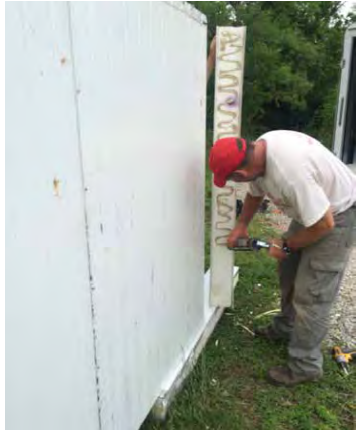
Figure 6. The panels are assembled with construction adhesive and self-tapping screws at the tongue-and-groove joints.
