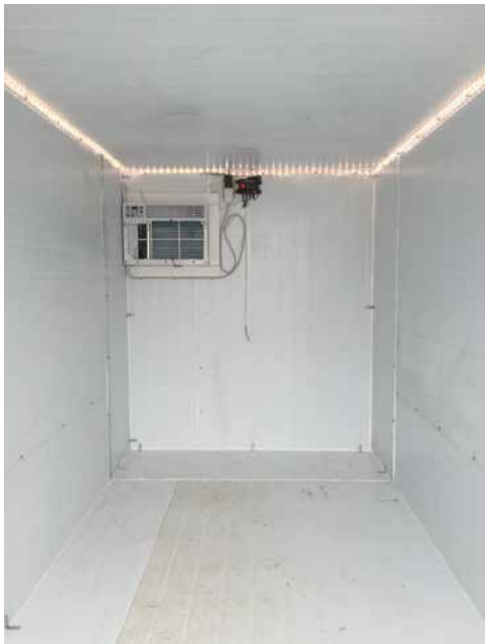
Figure 12. The trailer with cooling and lighting installed.
